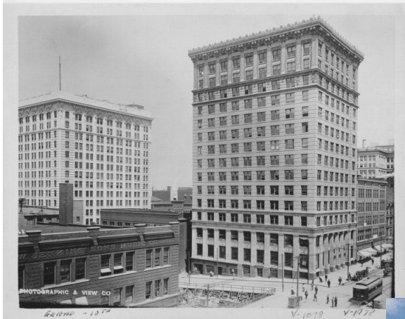
R.A. Long Building – James J. Lynn’s company office – 928 Grand Ave., Kansas City, MO (northwest corner of Tenth and Grand Avenue).
